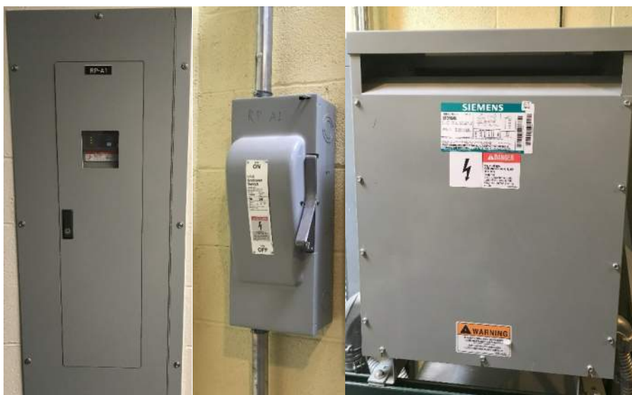
Photo 18: RP-A1 (Panel RP-A1, Disconnect, T-A1 respectively)
