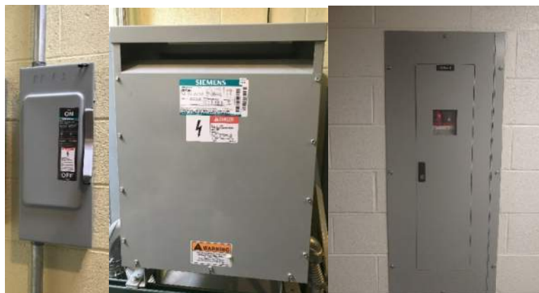
Photo 23: RP-F1 (Disconnect, T-A1, RP-F1 respectively)
