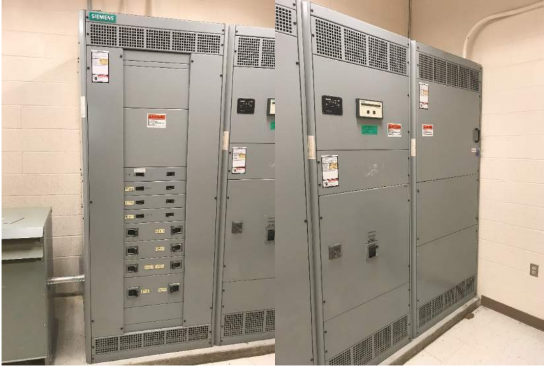
Photo 16: Main Switchboard
